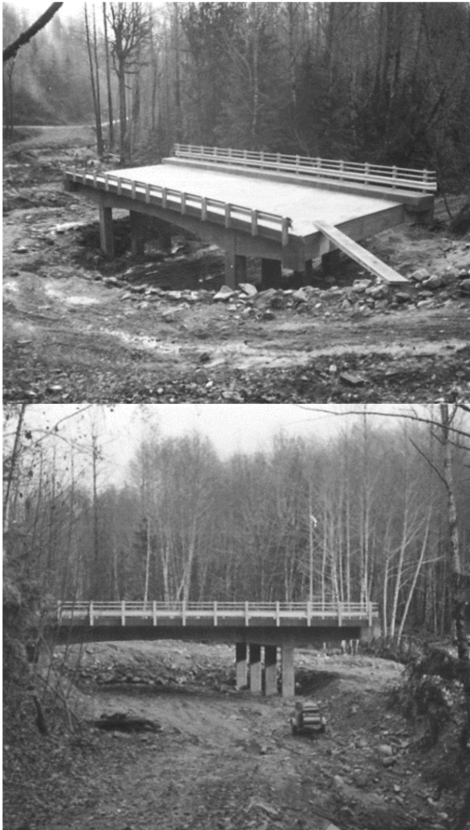
Figure 1-2 Views of Construction of Current Tenas Creek Bridge, Ca. November 1962 (from USFS)
